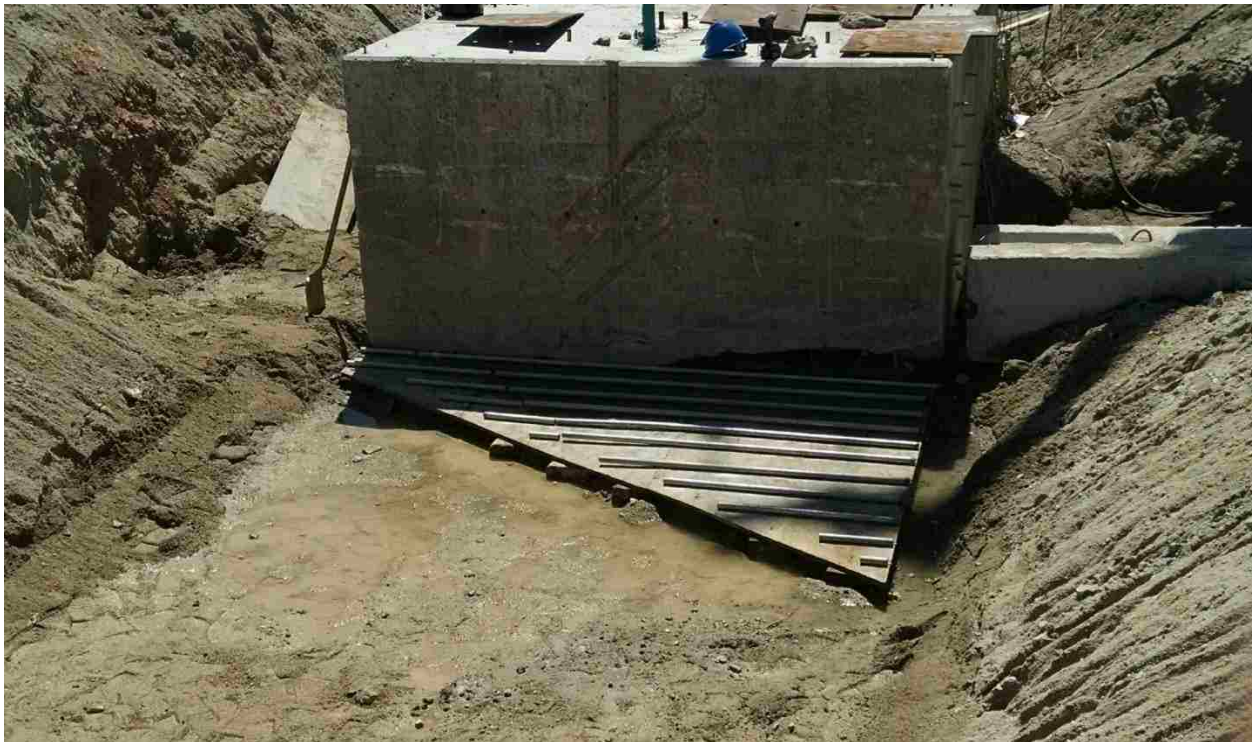
Figure 3-5: Skew wedge base composed of railroad ties, 0.75-inch plywood, and rollers
