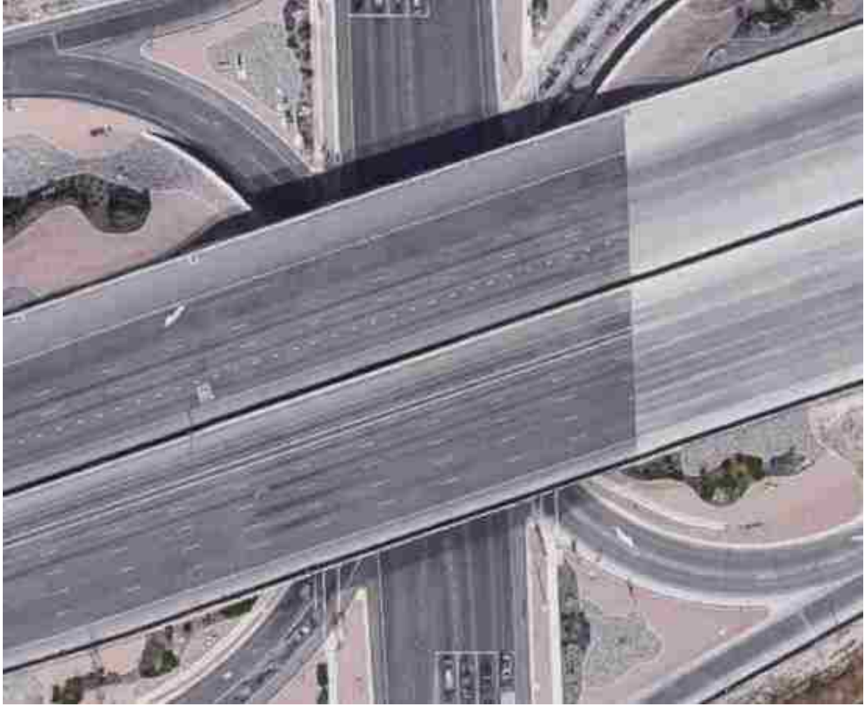
Figure 2-16: A wide skewed bridge located on Interstate-15 in Lehi, Utah (adapted from Google Earth)
